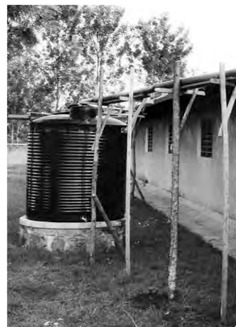
One of the TELD buildings, with a plastic water tank.
