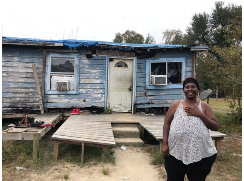
Lashon Turner's home was damaged by Hurricane Michael.
