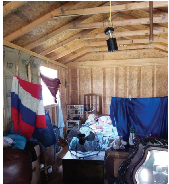
Ms. B's home before work began.
